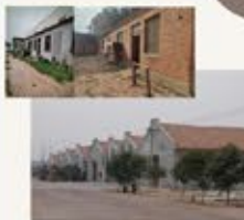
Original Appearance of Workshop
